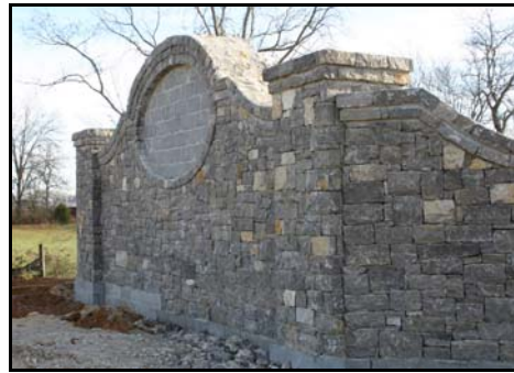
Williams Park entrance construction
